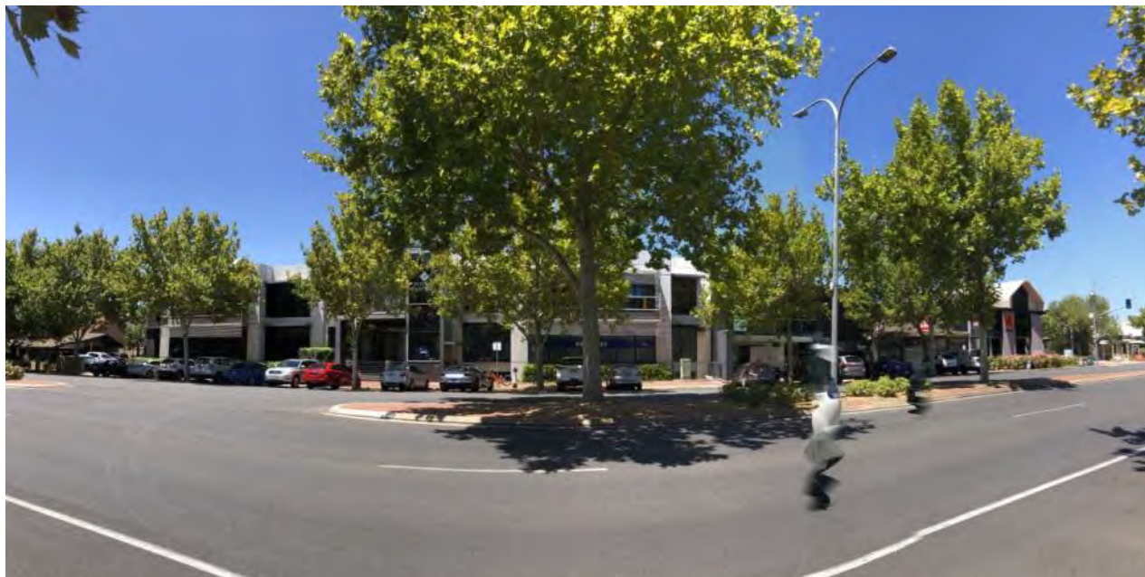
Recent modern office development on Hutt Street immediately west of the subject land.
